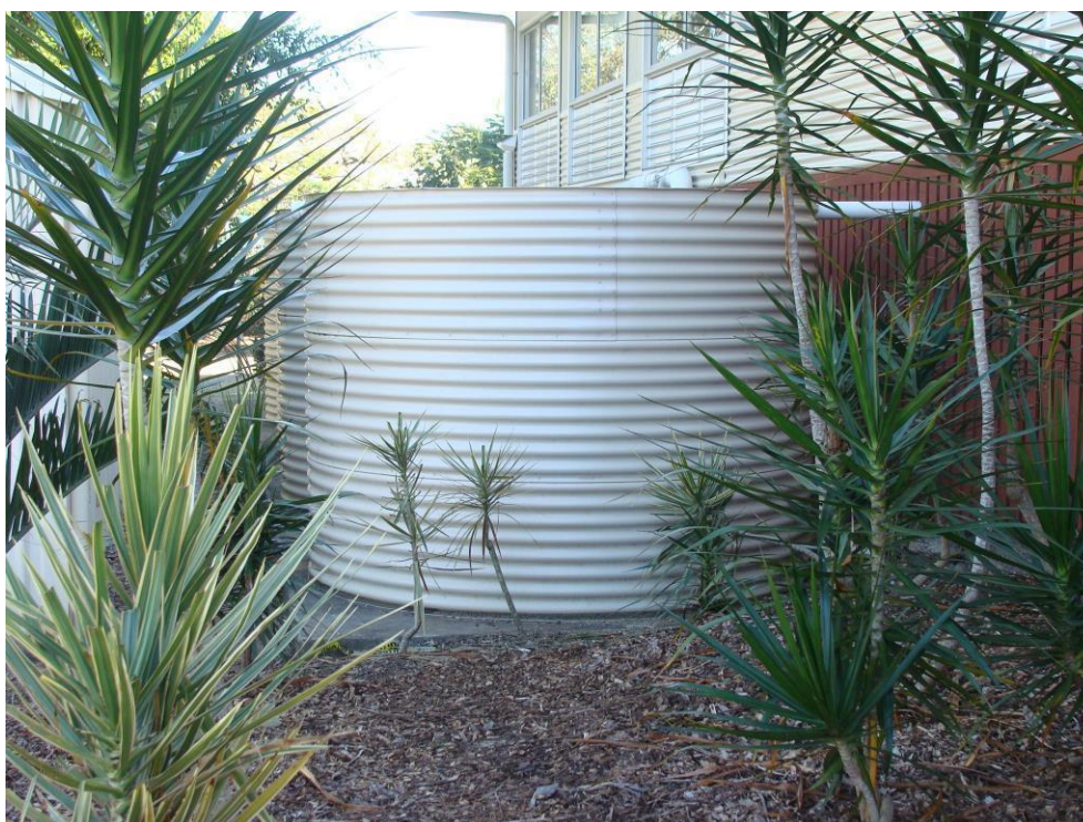
Figure 2: CHW and the Ballarat West PSP support rainwater tanks as an effective means of achieving potable water substitutions.
